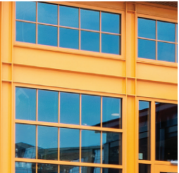
Punchy Color at Doors + Windows
