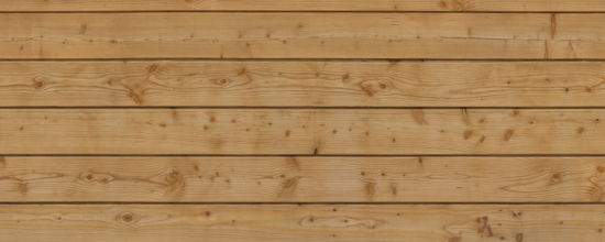
Stained / Painted Wood Cladding
