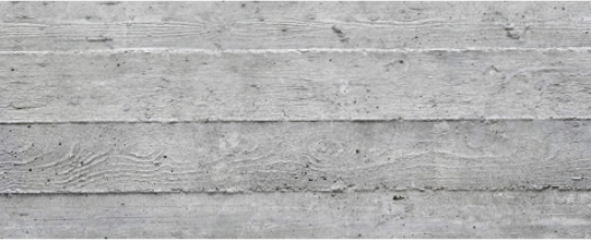
Board Formed Concrete
